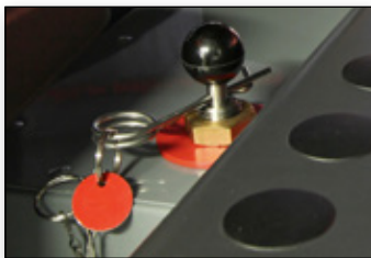
Manual fire extinguisher
